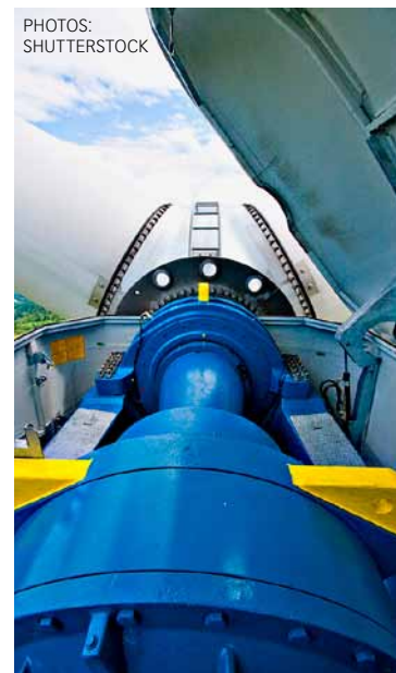
View of a windmill drivetrain from the top of the nacelle.
